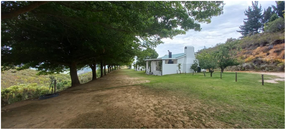
View of existing cottages and camping area
