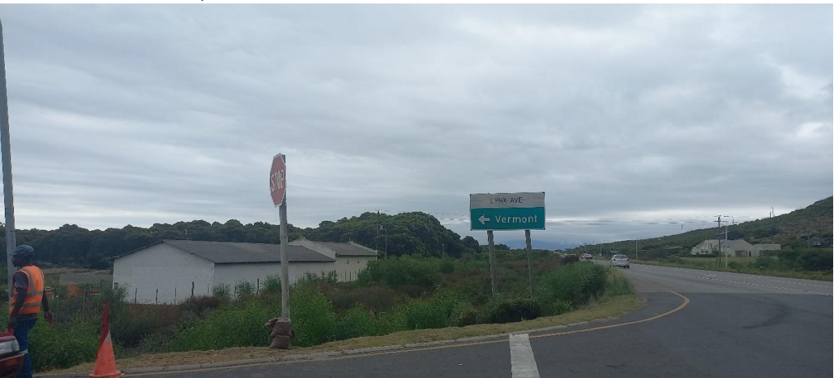
View of the site off the R43, corner of Lynx Road, looking towards the west. Building on site are derelict buildings on site (not older than 60 years)
