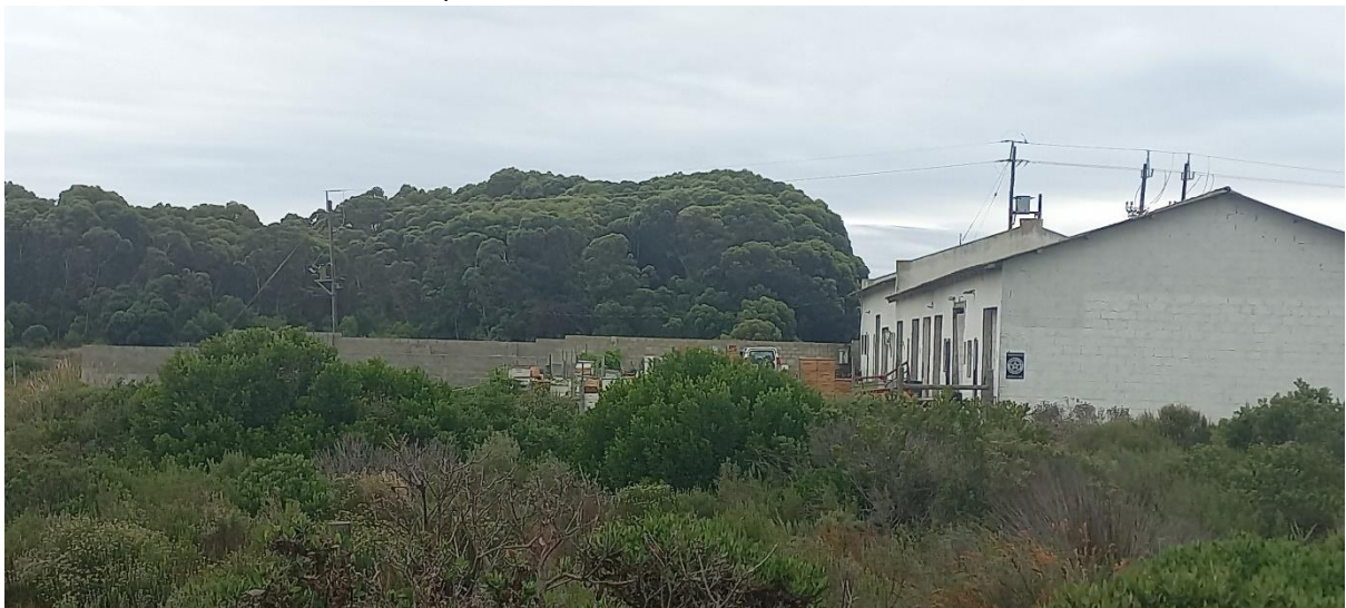
View of the site from the corner of Lynx Avenue and the R43
