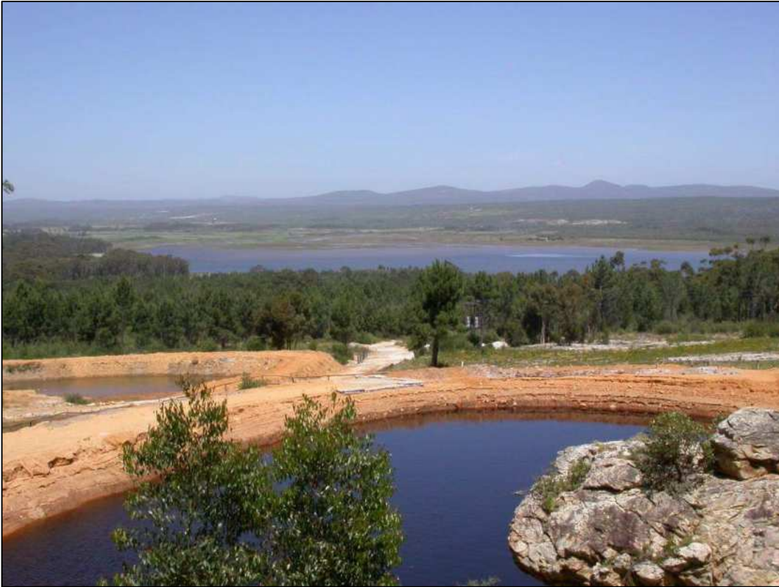
Photo 4. View of dams and infrastructure in site, looking towards the R43 and Kleinrivier (2012). Impacted areas, infrastructure and diversion of water evident in 2012.
