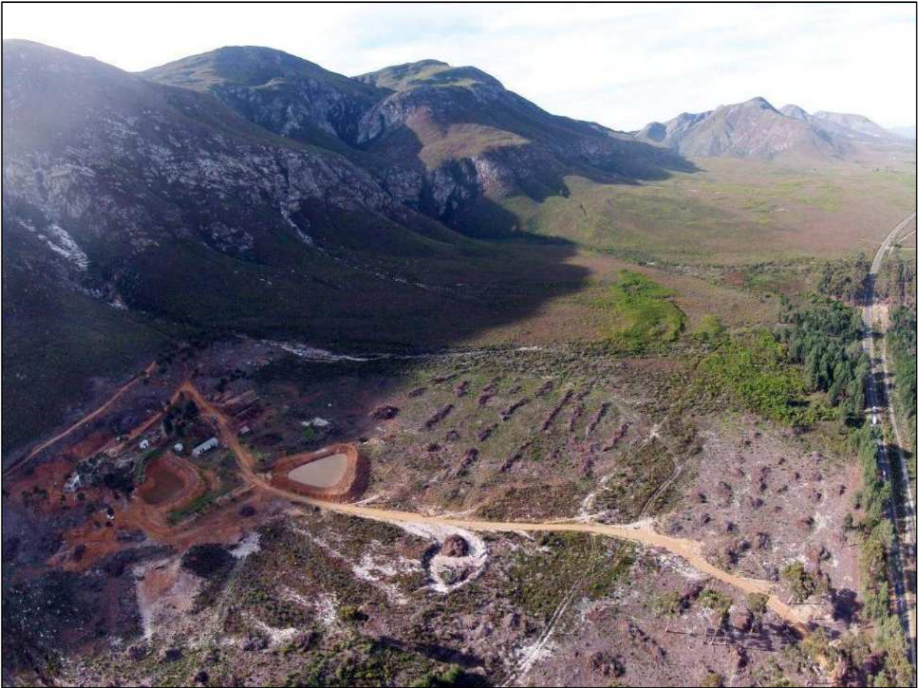
Photo 8. Aerial footage of the site 2012 – the property is extensively disturbed. Internal roads evident.
