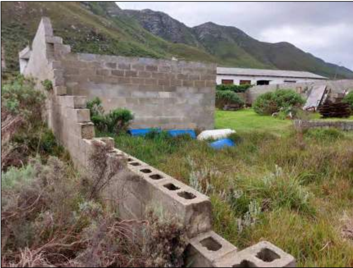
Figure 5-4: Derelict buildings located in the north of the proposed site.
