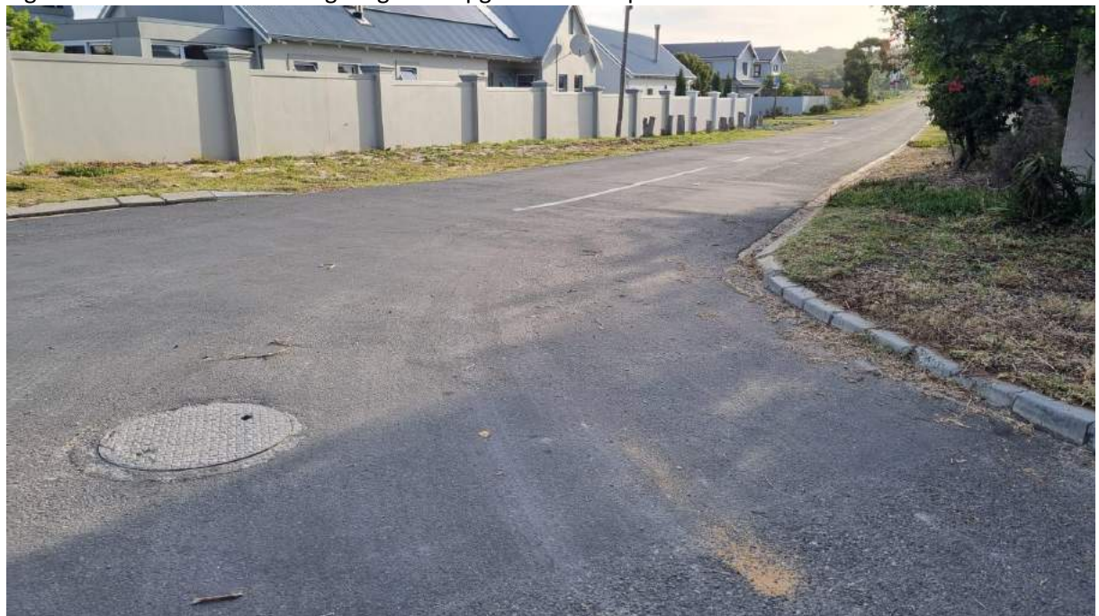
Figure 8.3 A. Manhole on existing pipeline along Malmok
