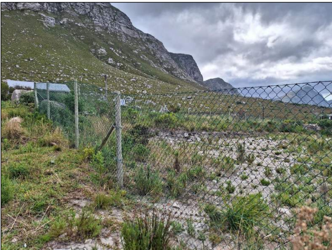
Photo 2: Clearance of vegetation with some bit of vegetation growing
