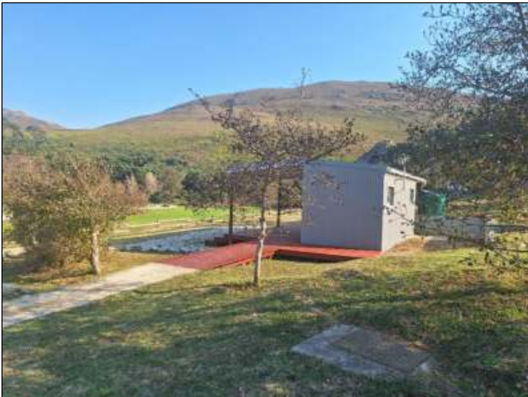
Photo 1: (Site 1) side view of the office developed on site that was cleared. The area did not contain indigenous vegetation and was characterised by lawn.
