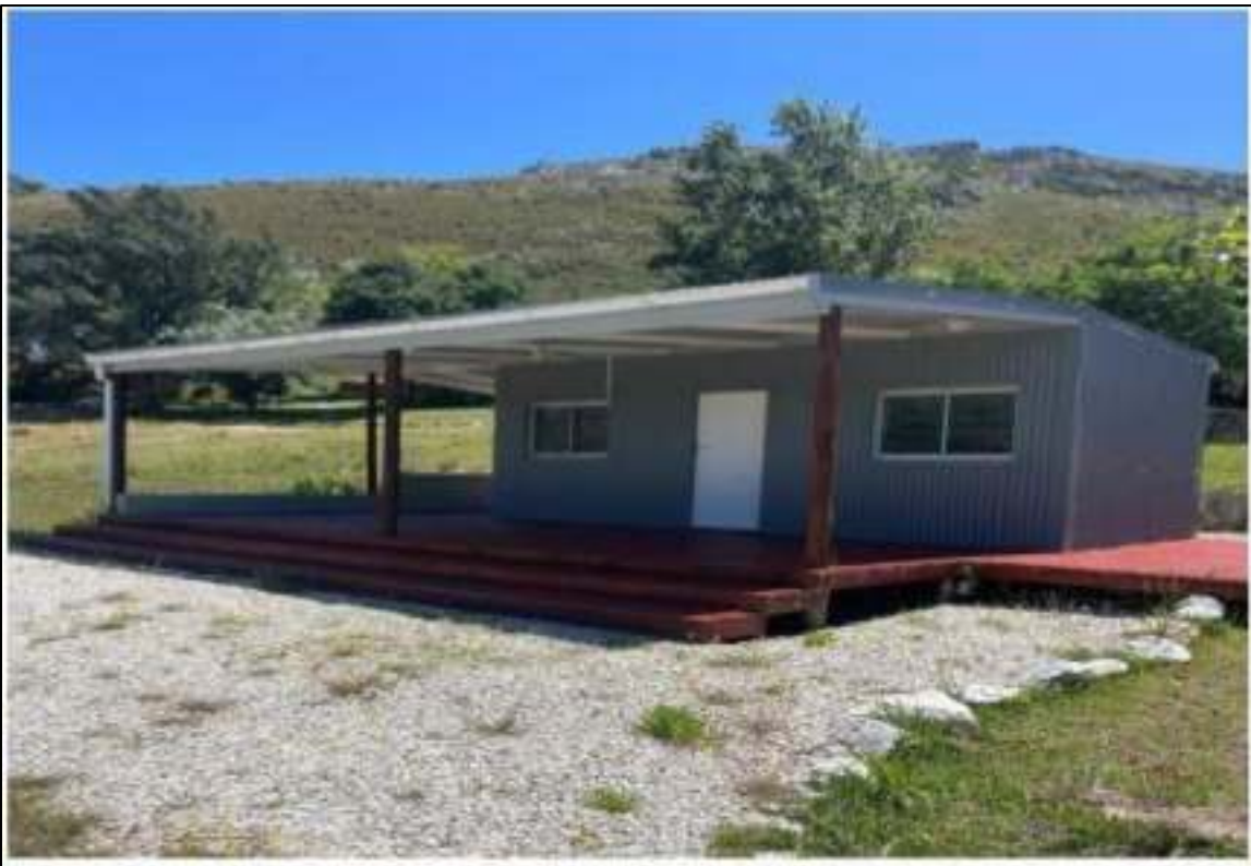
Photo 1: View of the site cleared in 2020 for the placement of a container in an area measuring approximately 133m 2 .
