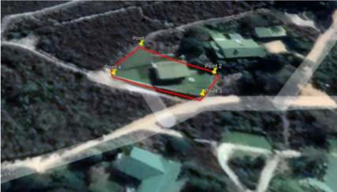
Figure 3: Aerial view of Site 2 showing approximately 534 m 2 of transformation.
