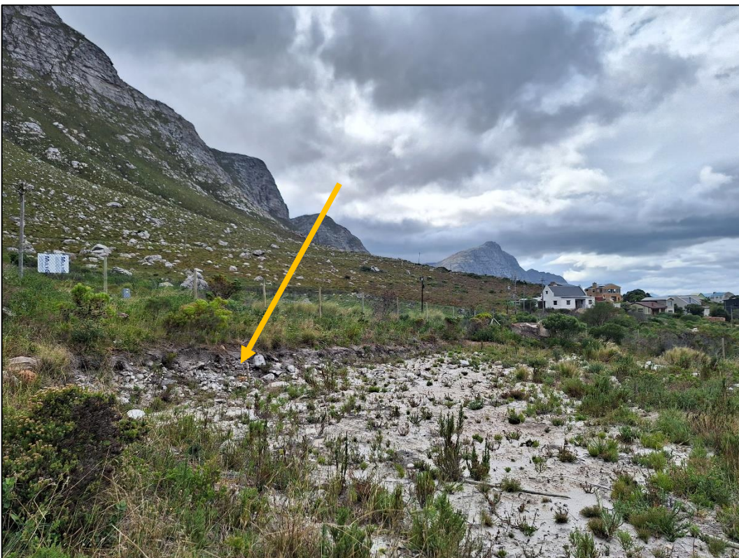
Photo 3: The image shows that excavation took place onsite.
