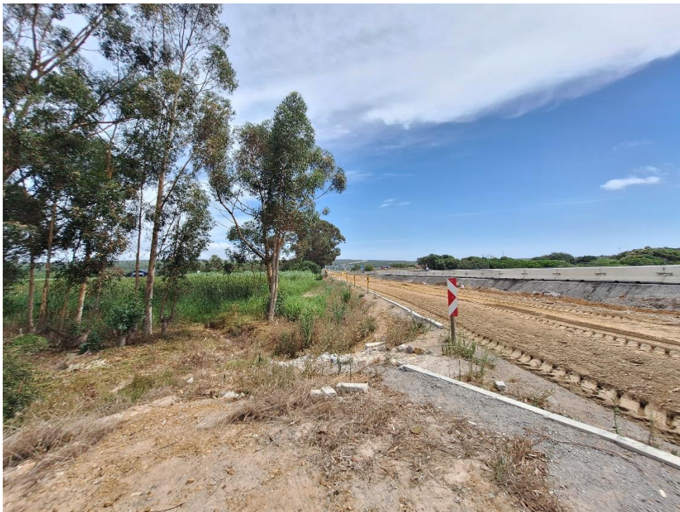
The R43 alongside the property (western boundary)
