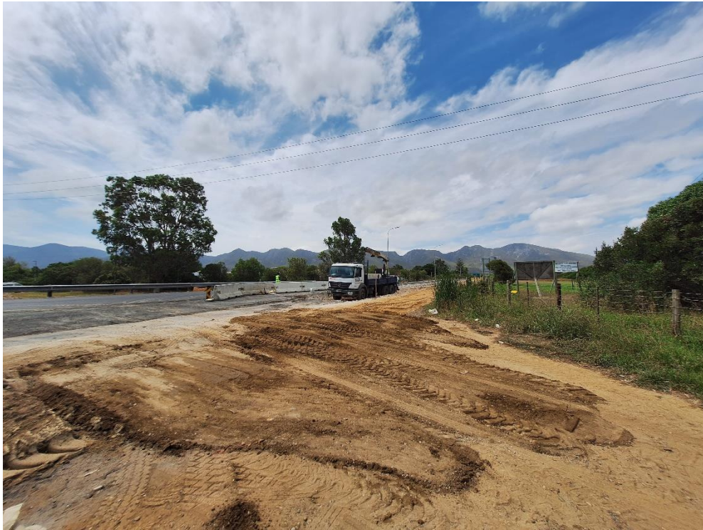
The R43 alongside the property (western boundary)
