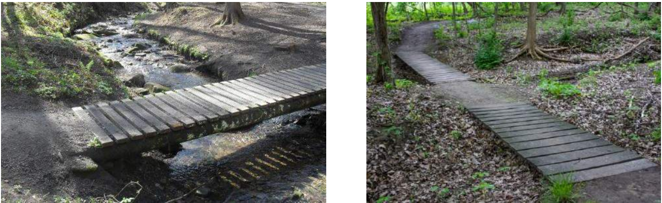
Figure 21. Bridges and boardwalks
