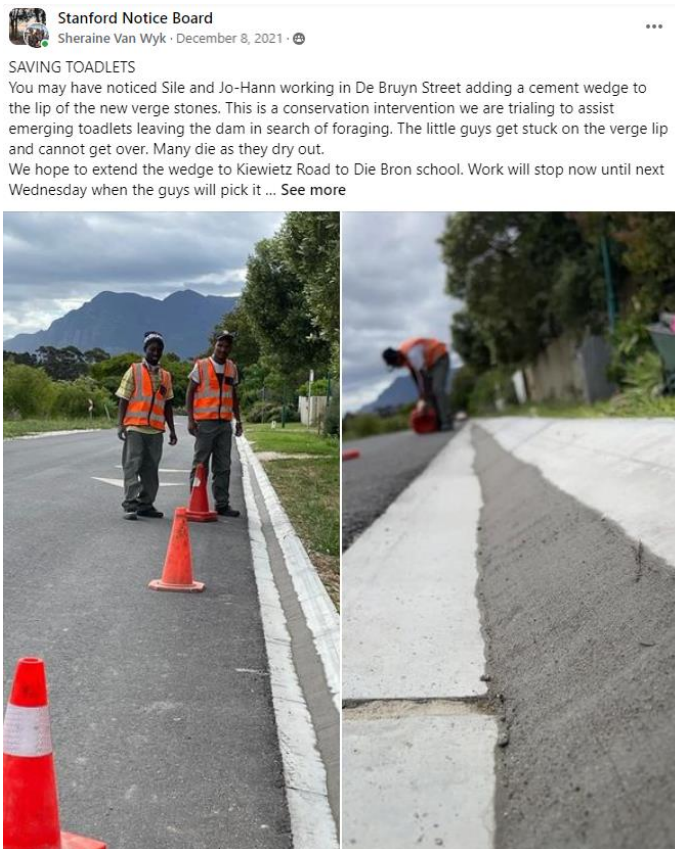
Figure 5: Filling the sharp edge of the verge stones to assist the safe passage of toadlets to their foraging grounds. [Source: Whale Coast Conservation Facebook Page, 8 December 2021]
