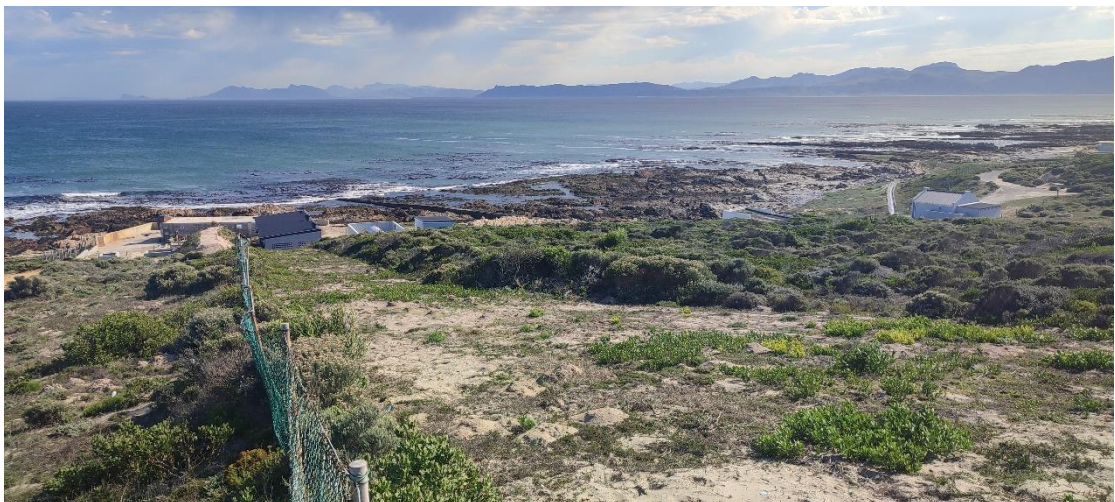
Plate 5: View west along proposed pipeline route to existing pumpstation, with brushcut area to the right (north) of the fence.
