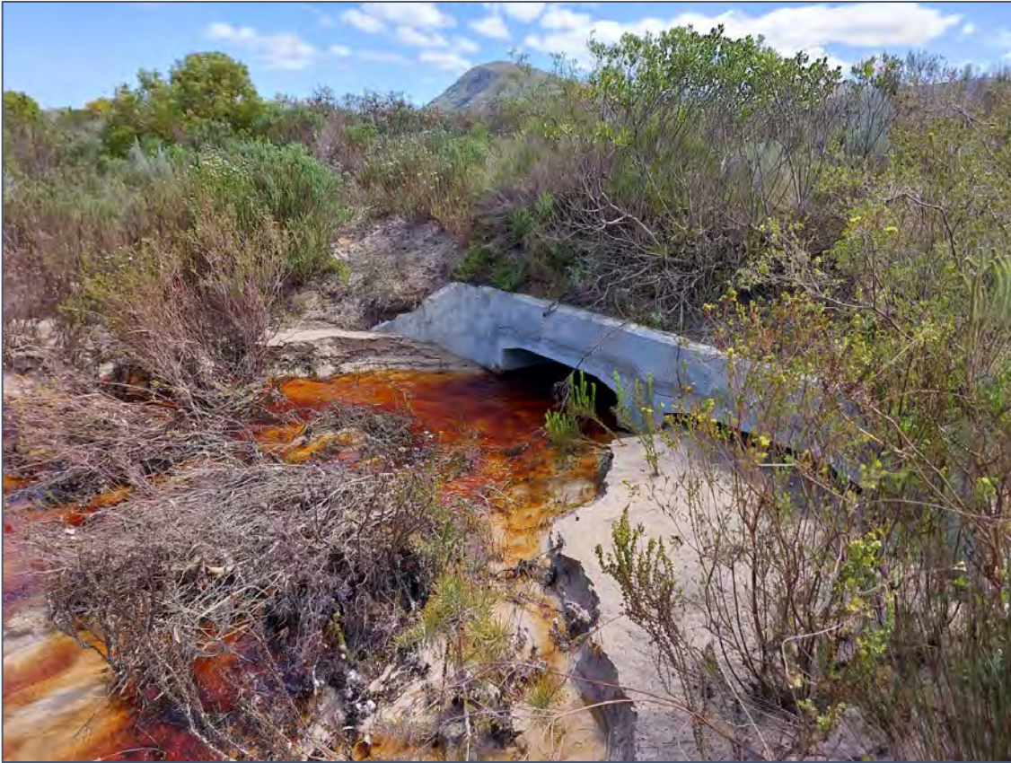
Figure 5-9: Culvert and SW flowing through the site.
