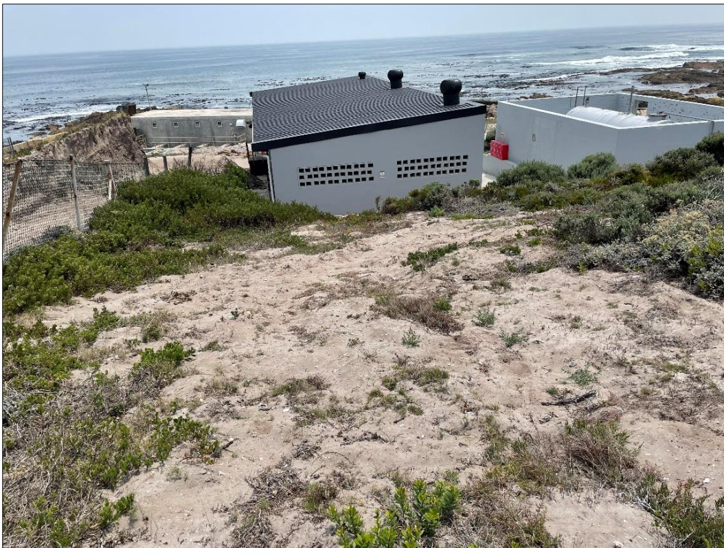
Figure 16. Site 088. The pumphouse is the building in the background of the plate.
