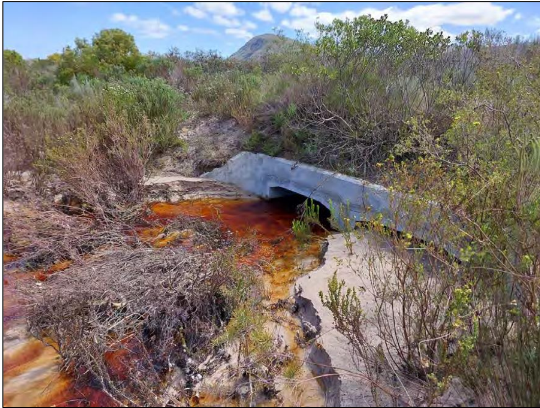
Figure 17: Culvert and stormwater flowing through the site
