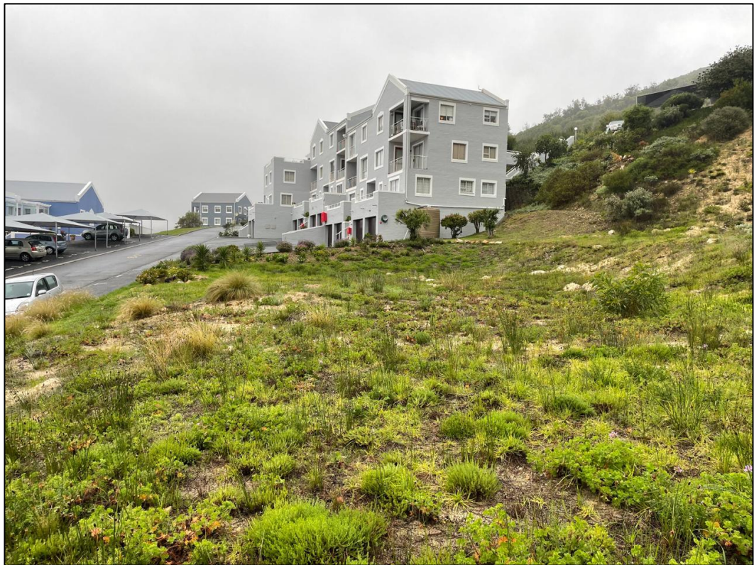
Photo 10. Showing the development area on site and adjacent existing activities
