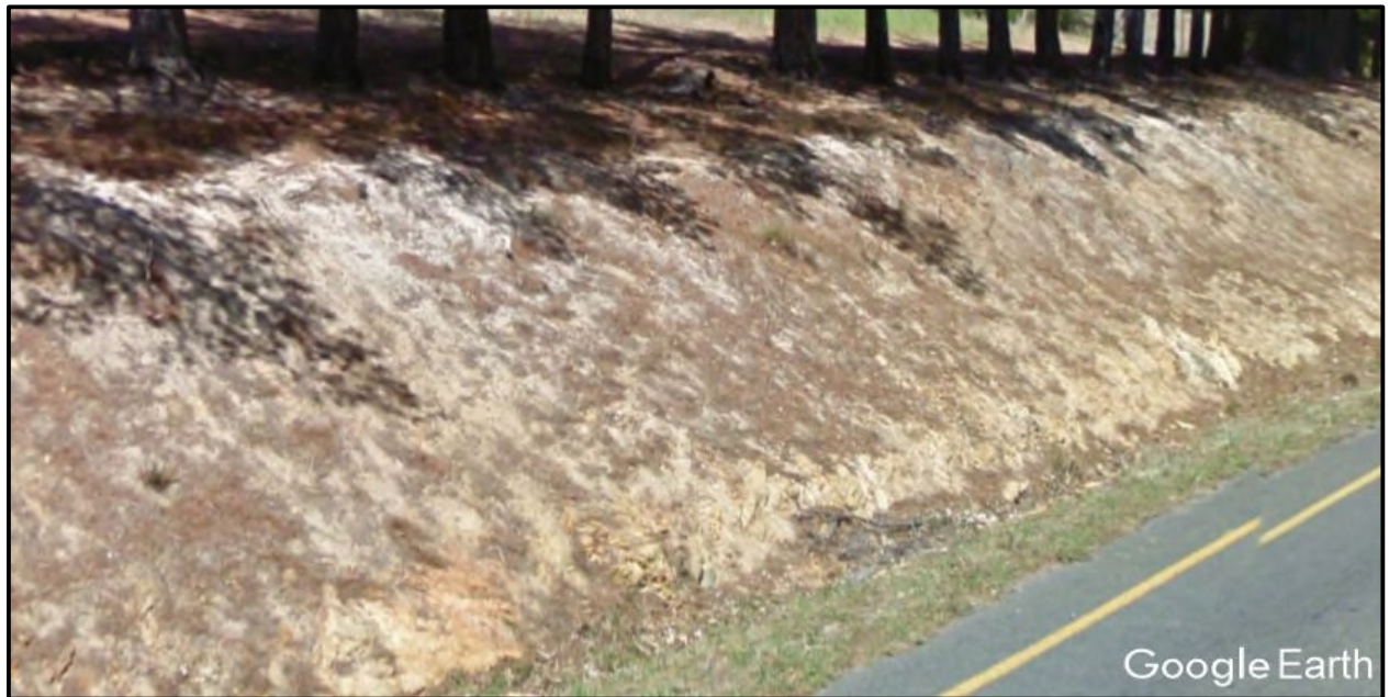
Figure 3. Road cutting near the development site showing the weathered Bokkeveld shales.
