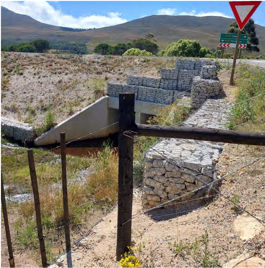
Figure 5-12: Hemel en Aarde Road and associated culvert.
