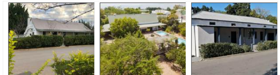
Figure 56: Variety of building sizes and erven, Britz 2024
