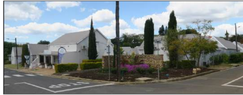
Figure 50: One of the few 'gated village/ retirement village' developments in the town.
