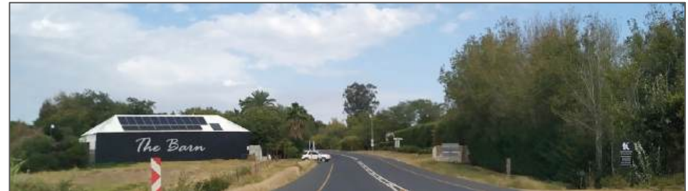
Figure 32: R311 Eastbound passing the lower/northern site (left)
