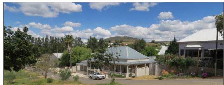
Figure 49: Typical scale, roofscape and development patterns
