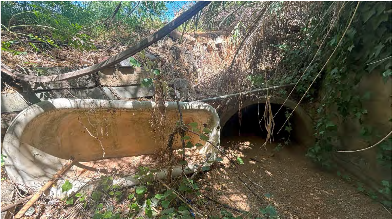
Figure 5-18: Point at which the Krom River emerges from the underground pipeline in the northern portion of the site. Rubble has been used for infill and bank stabilisation.
