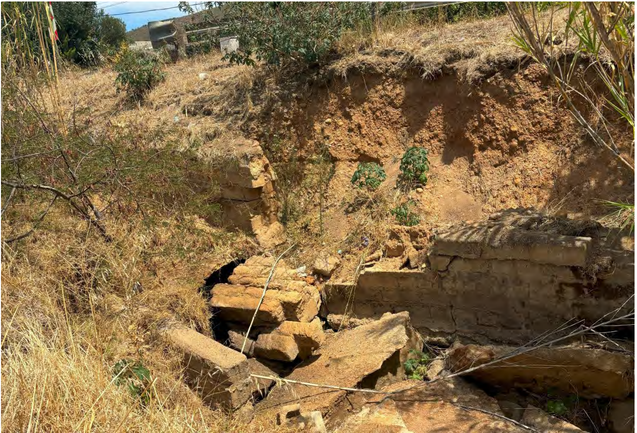
Figure 5-17: Point at which the Krom River enters the proposed development site by means of a degraded stormwater channel. Bank stabilisation measures have collapsed and are currently blocking the stormwater pipeline.
