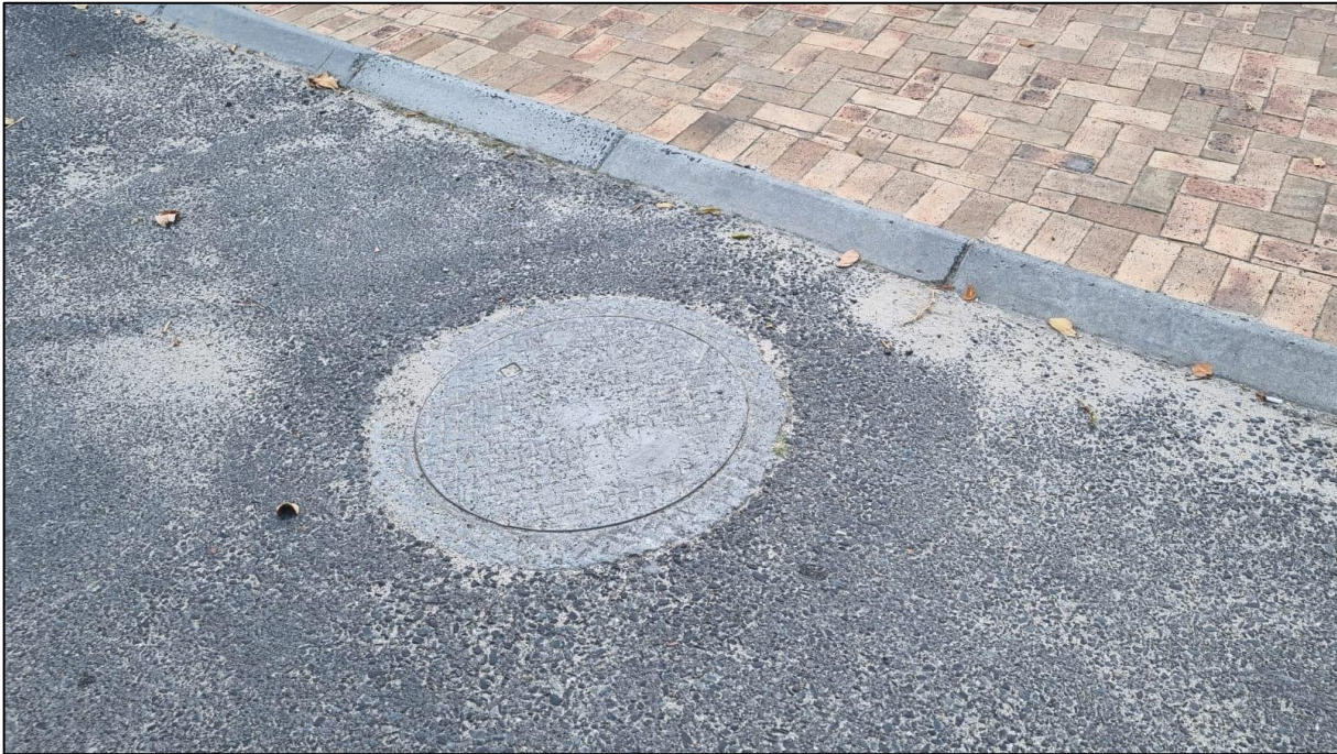
Figure 7.3-B - Manhole on existing pipeline along Kogans – upgrade required.
