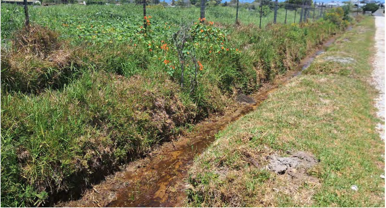
Figure 5-8: Channel along the access road, within the UVBW.
