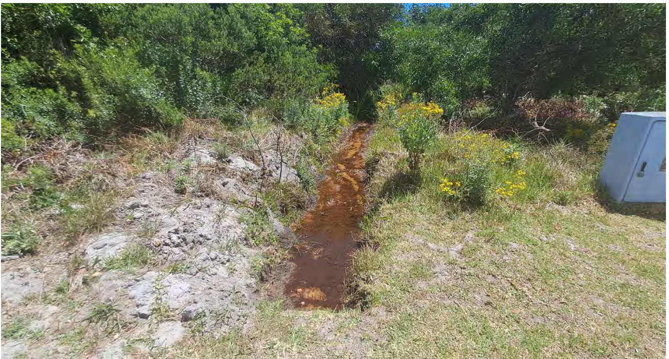
Figure 5-7: Channel within the UVBW, adjacent to the entrance / access road.
