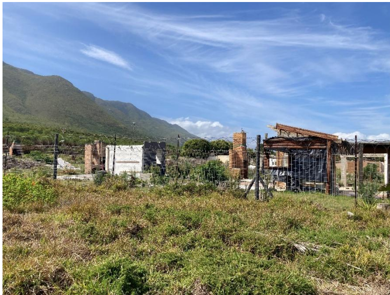
Photo 2. RE/1489 looking east ( Source: Lornay, 2025 )
