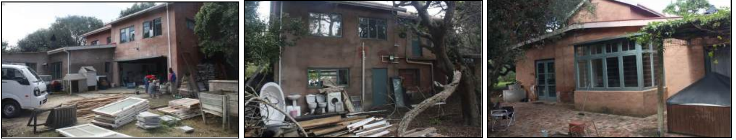
Figure 5.1 to 5.3. Existing residential structure on the property
