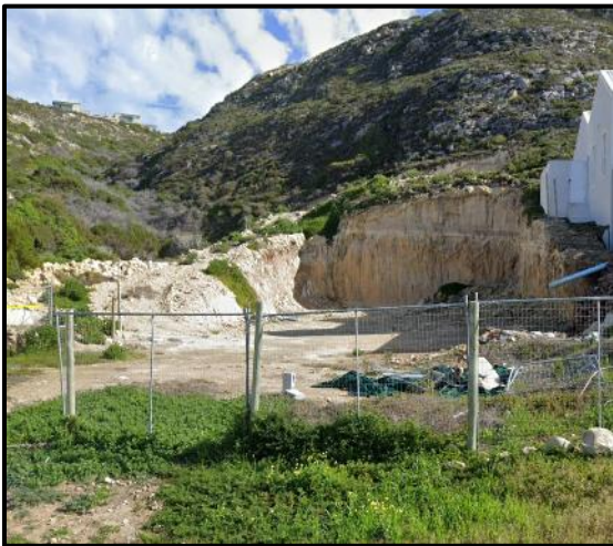
Figure 16 The gaping hole in Spookdraai. Photo: Courtesy Google Street View.
