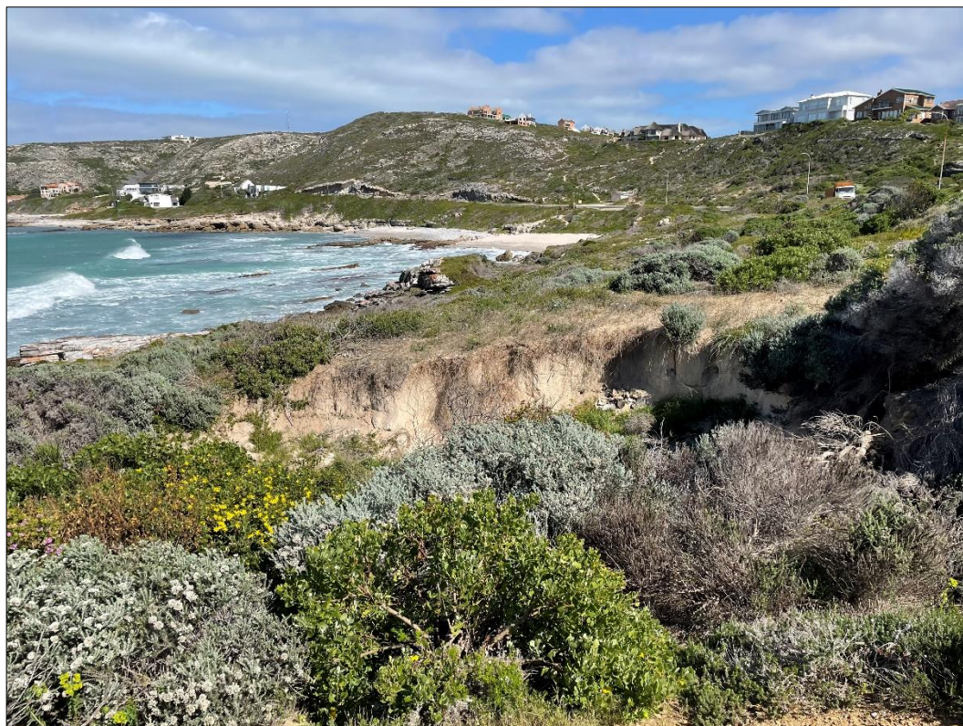
Figure 7. Deep donga in the foreground created by the stormwater outlet. View facing southwest.
