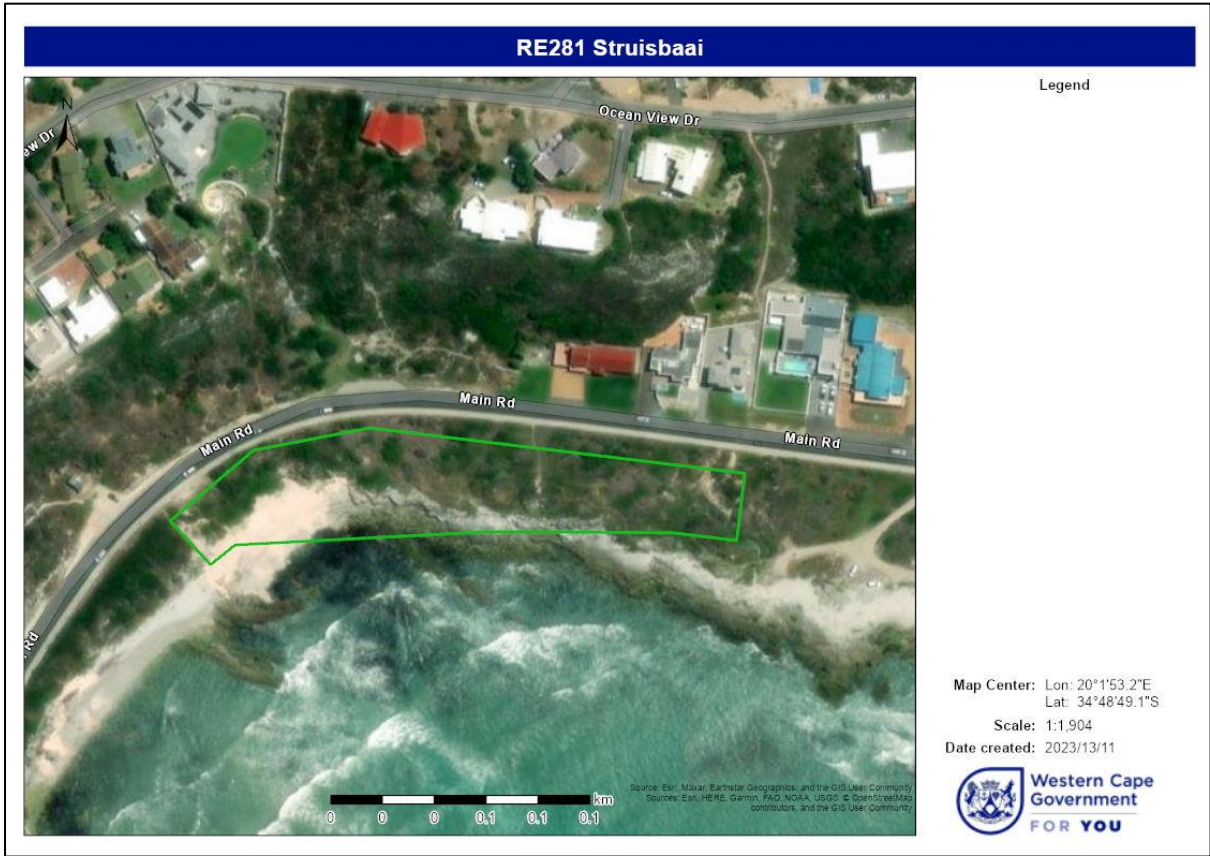
Figure 4. Aerial view of subject property
