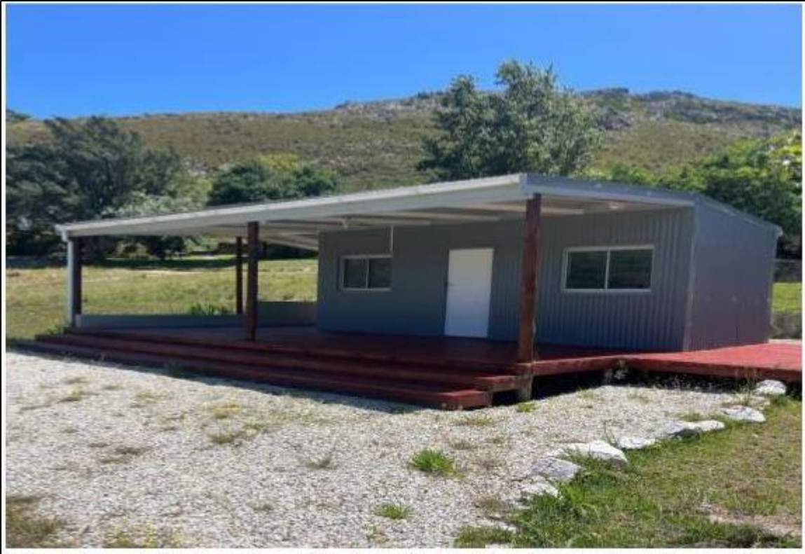
Photo 8: View of the site cleared in 2020 for the placement of a container in an area measuring approximately 133m 2 .
