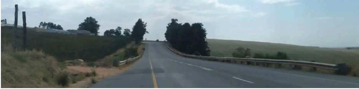
Photograph 4-15: R311 Westbound exiting western Riebeek-Kasteel.
