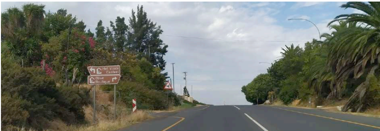
Photograph 4-32: R311 Eastbound approaching Het Vlock Casteel and the R46 intersection.
