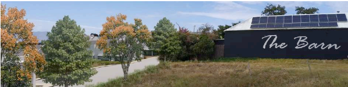
Photomontage 5-3 (Photograph 4–10): View of the lower site (south) and upper site behind from the R311.
