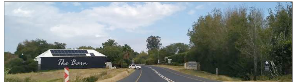
Figure 28: R311 Eastbound passing the lower/northern site (left)
