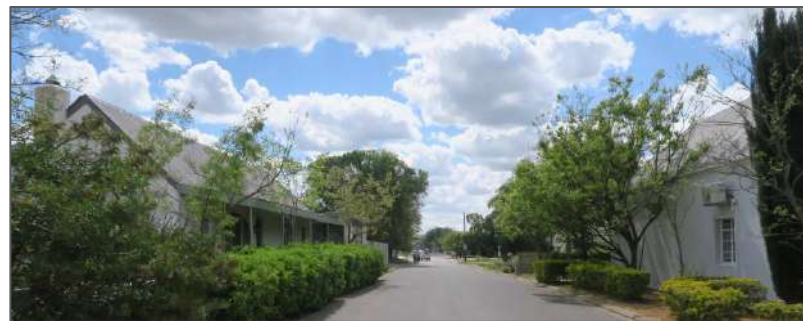
Figure 41: Typical scale, roofscape and development patterns
