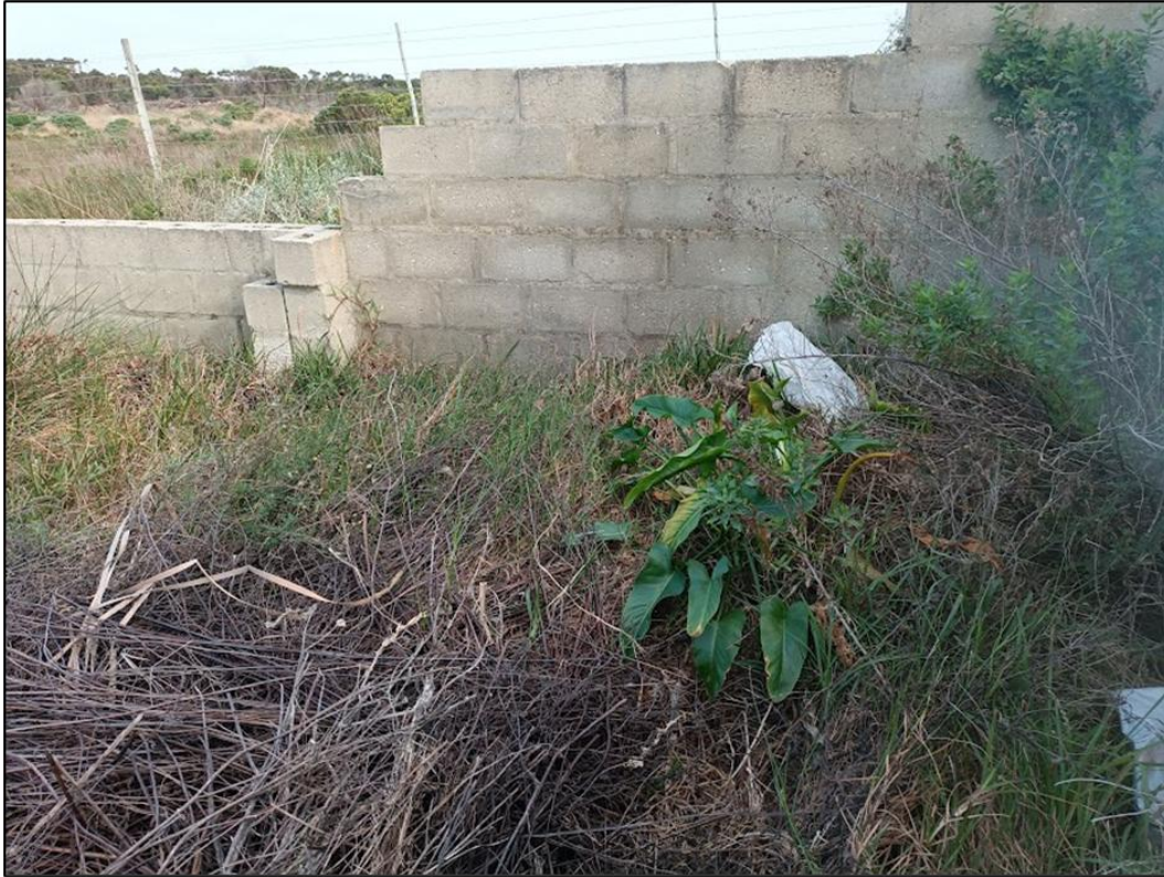
Figure 11e: Zantedeschia aethiopica growing alongside a partially demolished wall near the existing building on the site. Source: (EnviroSwift, 2025).
