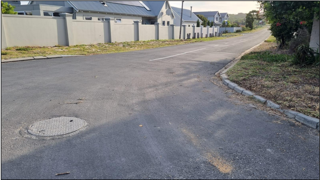
Figure 7.3-A. Manhole on existing pipeline along Malmok.
