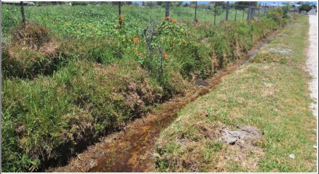
Photo 3: Stormwater channel along the access road which will be upgraded, within the UVB wetland.
