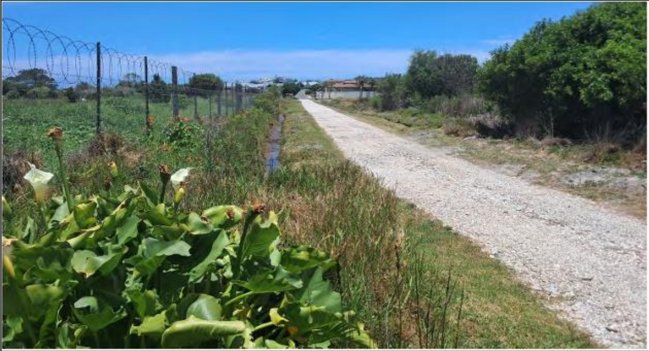
Photo 1: The existing access road that will be upgraded.
