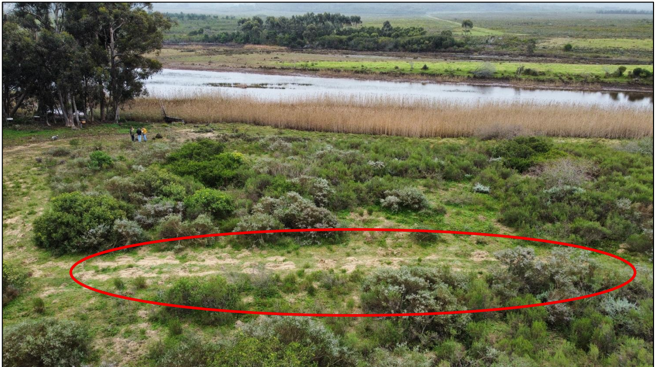
Photo 4. Overview of the existing access road. House 1 will be concentrated here which will connect both house 1 and House 2 access.
