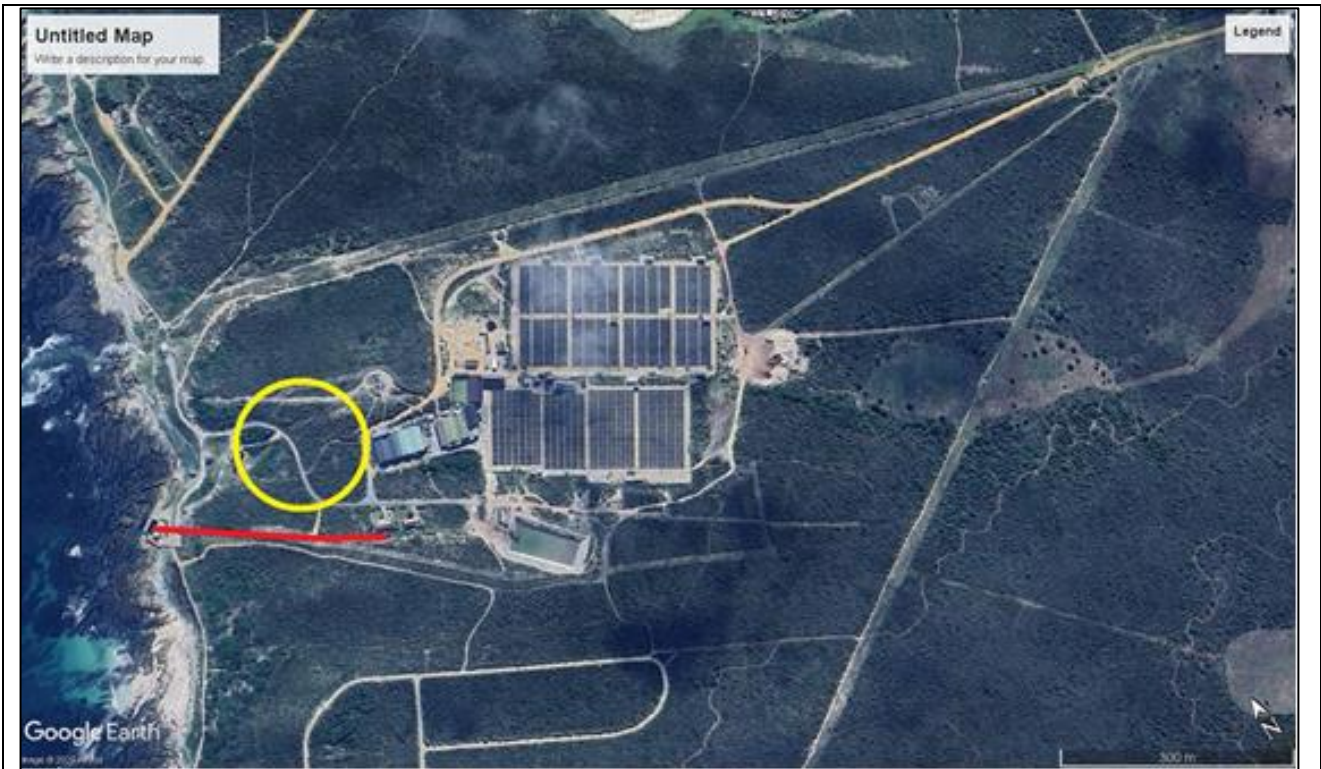
Figure 10: The pipeline corridor is indicated in red and the yellow circle indicates the limestone vegetation area.
