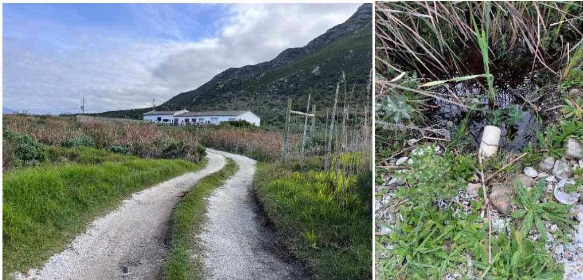
Figure 3.13: Images showing the entrance road from Lynx Road to the main dwelling on erf 1486 (left). This road contains numerous pipes to allow water to flow underneath it.
