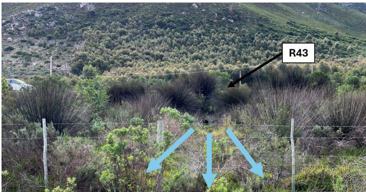
Figure 3.16: Image of a stormwater culvert underneath the R43 draining the upper catchment and discharging flows towards erf 1486.
