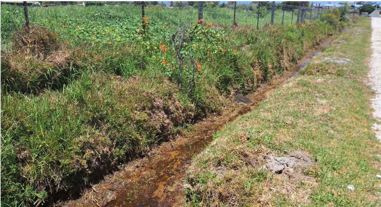
Figure 5-8: Stormwater channel along the access road which will be upgraded, within the UVB wetland.
