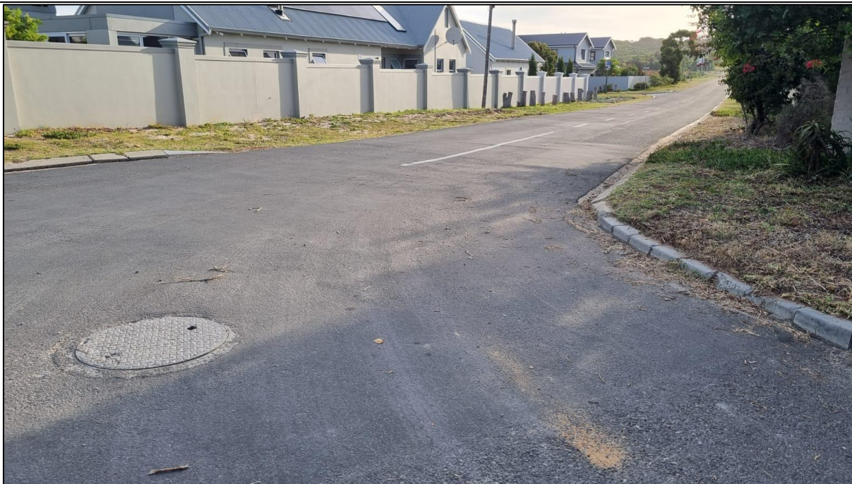
Figure 7.3-A. Manhole on existing pipeline along Malmok.
