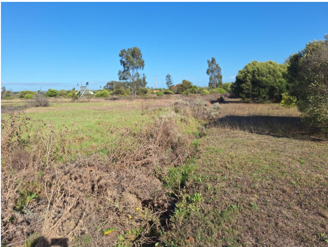
Photo 2. Site on the Western boundary – man made stormwater drainage ditch which links to the stormwater on the road.
