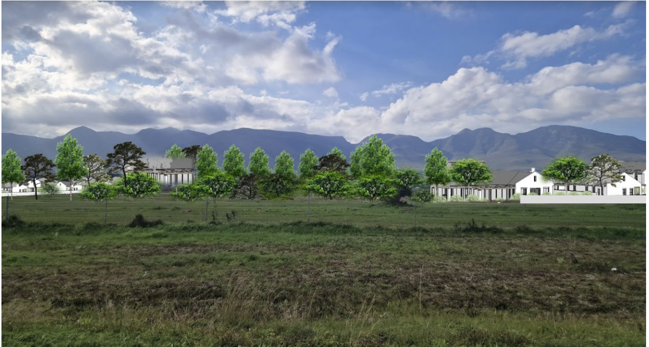
View 8: View from the R362 looking towards the site, view from the side of the road - visible, with high visual impact. Note the green area associated with the landscape plan of the development. Note that erf 1197 works in relation to this open area to create this embedded effect.
